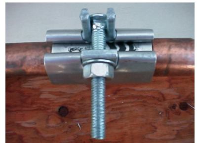
Retighten after 20 minutes...Leak is stopped!
